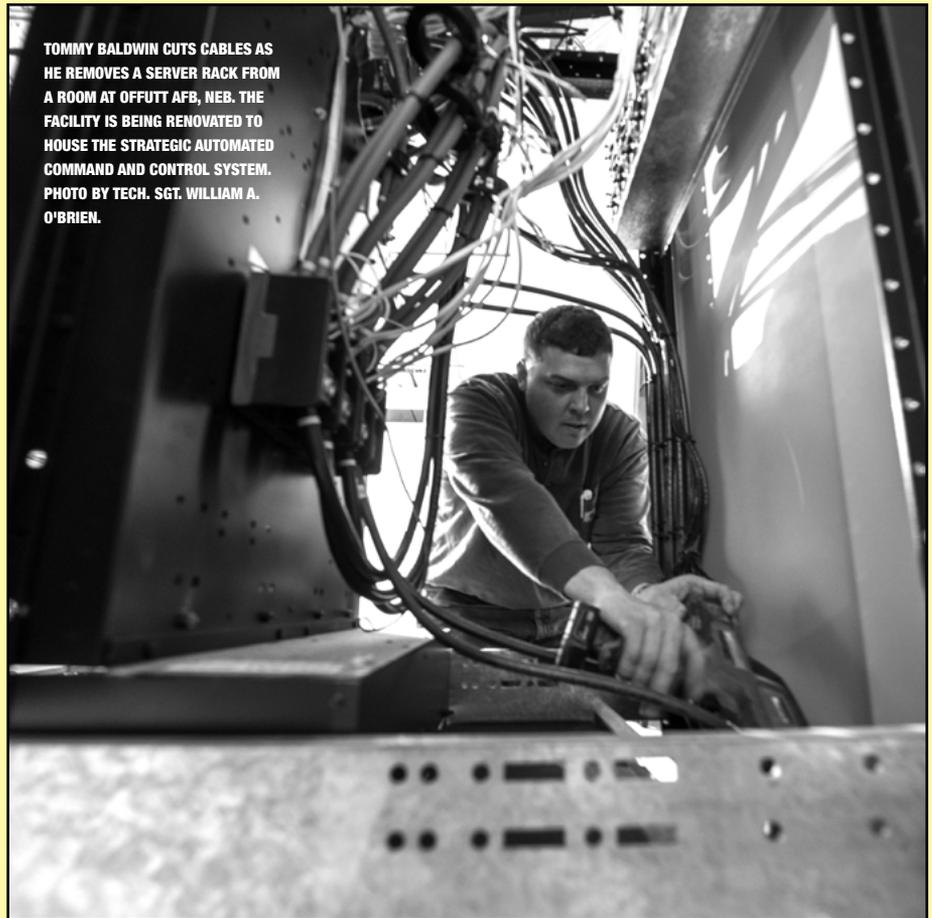
TOMMY BALDWIN CUTS CABLES AS HE REMOVES A SERVER RACK FROM A ROOM AT OFFUTT AFB, NEB. THE FACILITY IS BEING RENOVATED TO HOUSE THE STRATEGIC AUTOMATED COMMAND AND CONTROL SYSTEM. PHOTO BY TECH. SGT. WILLIAM A. O'BRIEN.
